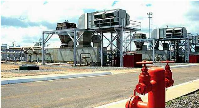
Figure 2. Air Inlet System with Filter and Silencer for a Gas Turbine Installation.
