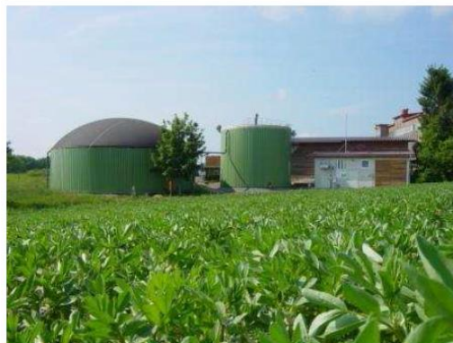
Fig. 6 Vertical digester in Germany, processing pig and poultry manure and crop silage
