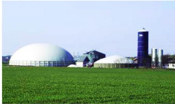
Fig. 5 Picture of farm scale biogas plant in Denmark, co-digesting animal slurries and energy crops (GROENGAS A/S)
